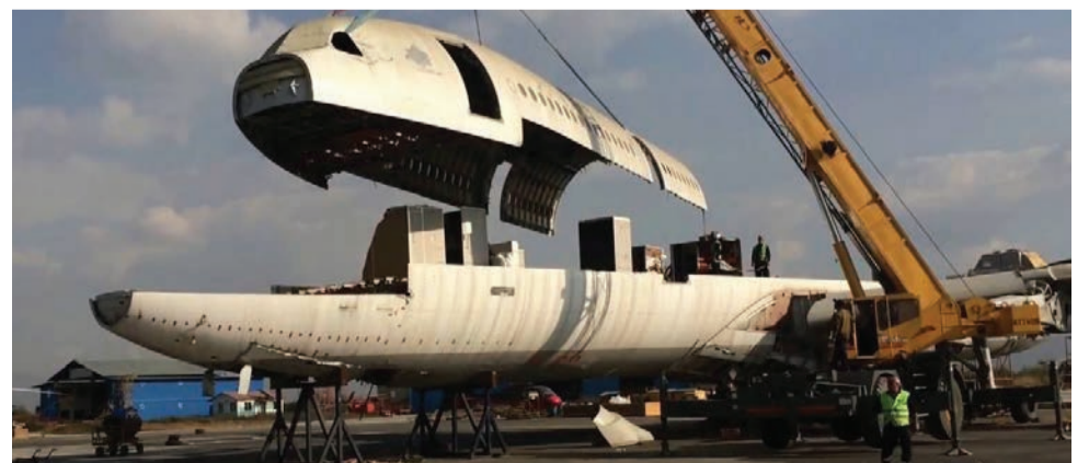
▲ Airbus A330-300 series costing USD 253,000,000 being dismantled.
