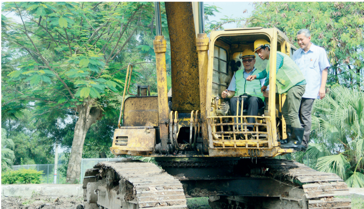
Izham manoeuvres an excavator at the Bandar Puteri reservoir on November 19
